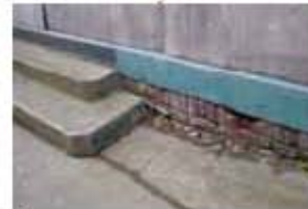
i) brick structure supporting concrete slab
