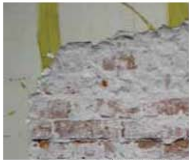
a) brick wall with plaster
