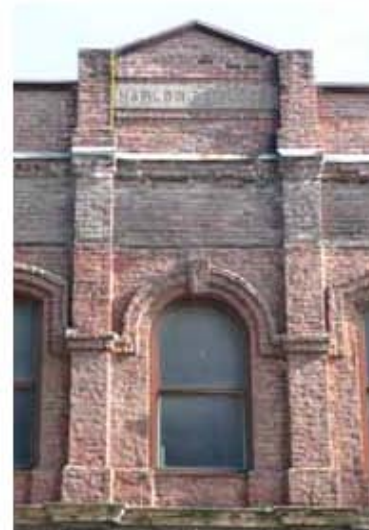
d) entry marked by plasters and small pediment
