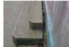
j) concrete steps leading to storefront
