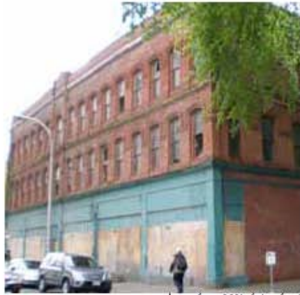
a) view from NW of storefront
