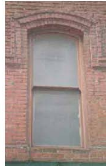
e) typical exterior window of hotel room
